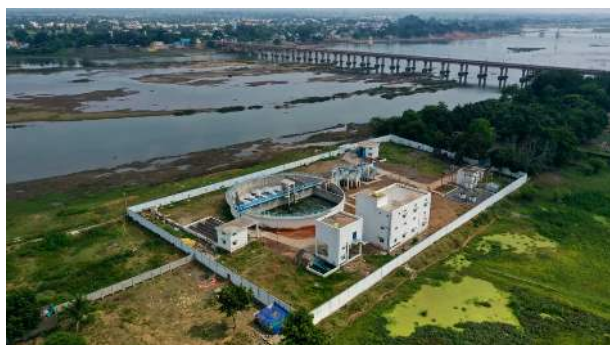
Photo: 7.6 MLD STP on Mahanadi River
